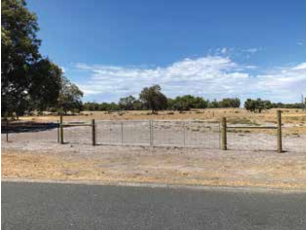
Gates installed at the Whiteman Park site.
