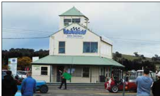
The Wakefield Park control tower with the dummy grid in the foreground
