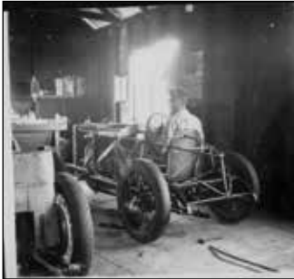
Fred James built this Morris Minor Special to race at Albany in the 1930s. The body shell used cane clad in canvas.
