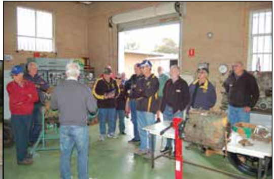
Ron Fabry (back to the camera) explains the vintage workshop set up in the generator room of the Department of Defence installation.
