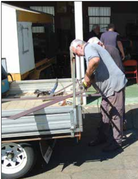
Glynn cutting steel plate to size
