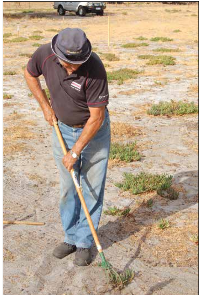
Ross Oxwell putting his words into practice at the building site in Whiteman Park
