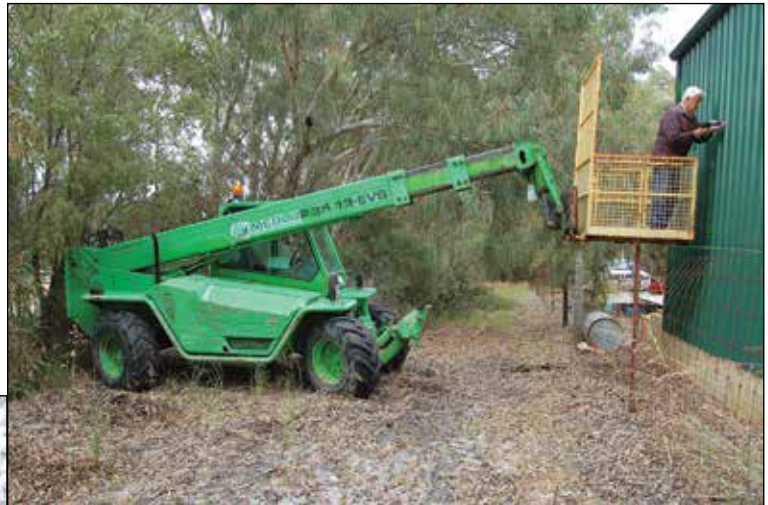
Above: Barry Mackintosh accepts a lift from Neville's telehandler to remove the bolts holding the shed together.
