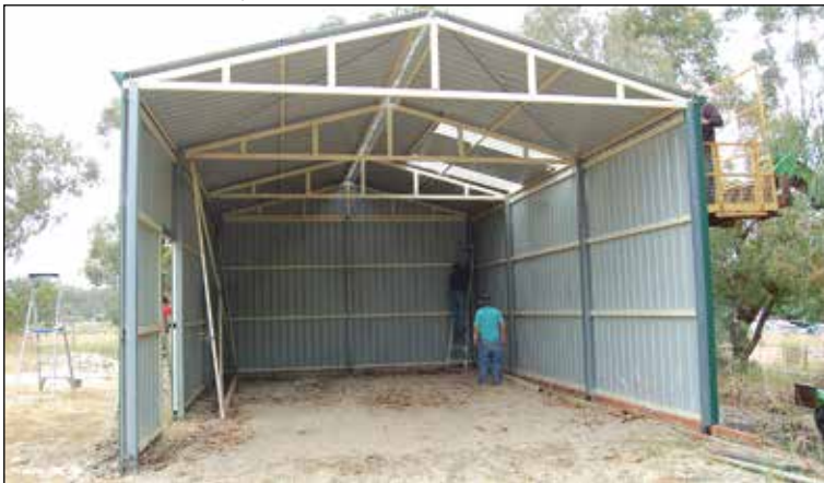
Above: Barry Mackintosh accepts a lift from Neville's telehandler to remove the bolts holding the shed together.
