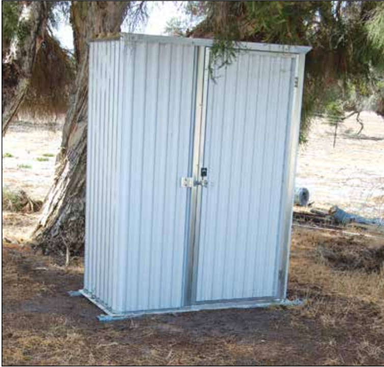
The site toilet, constructed from a small garden shed kit with a translucent fibreglass roof in place of the standard galvanised iron roof to avoid that 'black hole' feeling for occupants.
