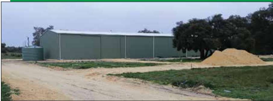
The new clubrooms with water tank and 60 tonnes of road-base.
