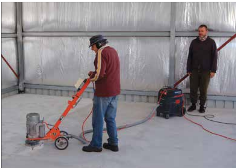
Ross Oxwell mans the grinder while Chad Raven monitors the vacuum cleaner, on the clubroom floor
